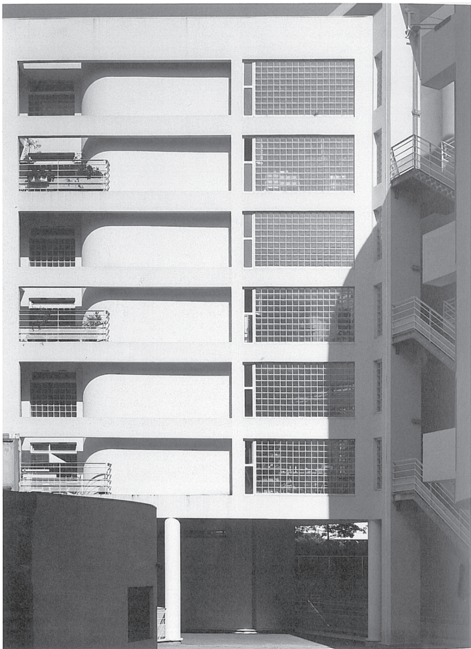
East wall of A-wing
