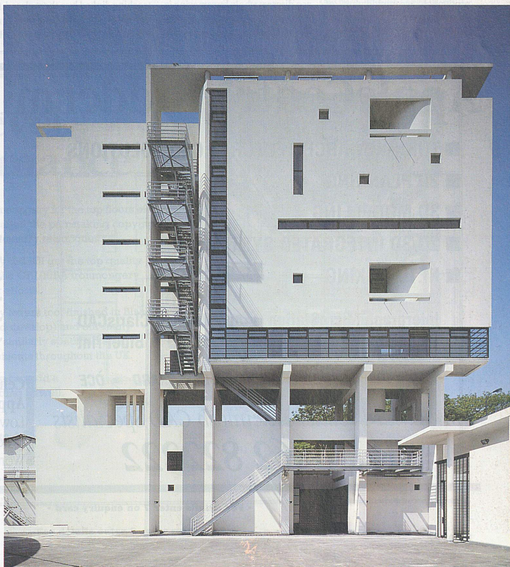
Top right Link across the north side of the courtyard to the service building.
