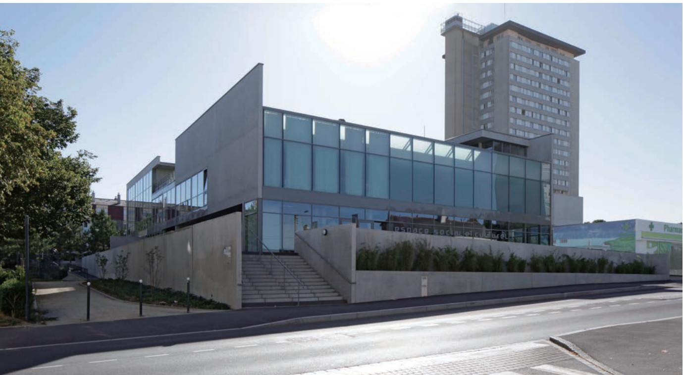
West elevation on the Louis et Rene Moine Street
