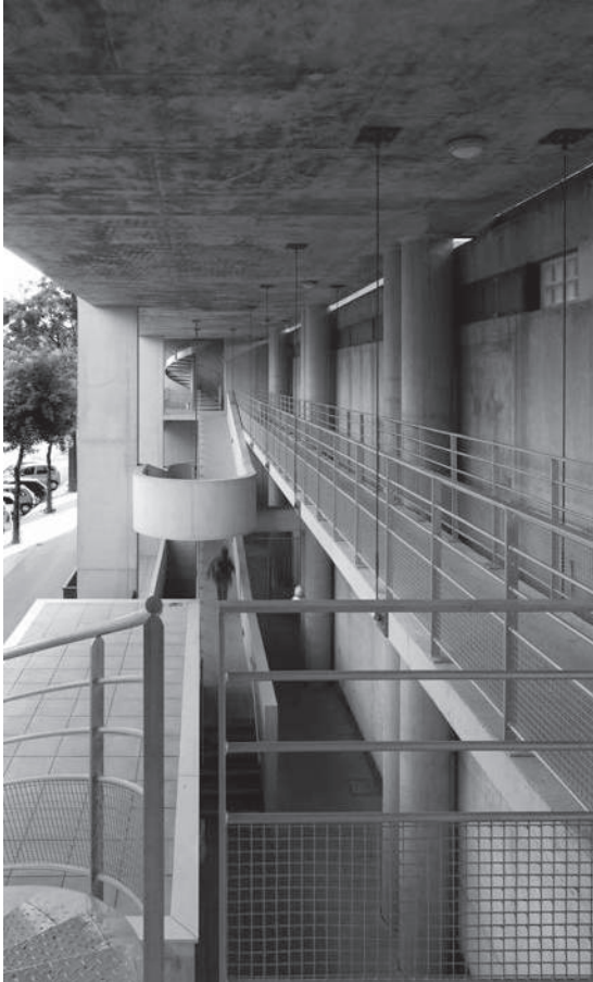
View of the pedestrian ramp under the pilotis
