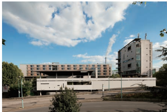
View of north-west elevation from technical and administrative center tower
