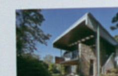
The Creek House Australia 498
