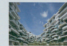
'UNIK' Apartments France 550
