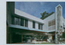
Corner House Australia 532
