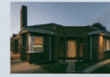
Clerestory House Australia 544
